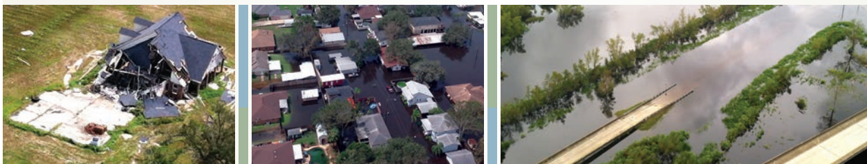
Hurricane Isaac had Category 1 sustained winds but extensive damage from flooding on I-10 in LaPlace.
